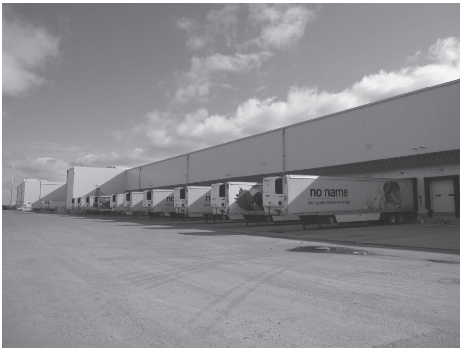
Photo 5.2 Grocery chain cold storage facility, Regina, Saskatchewan
